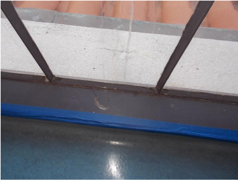
EW4. Southeast wing second floor corridor.
