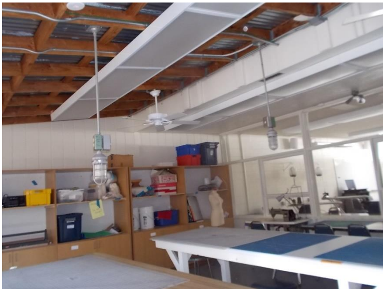
R3. Enclosed patio; underside of exposed roof structure.
