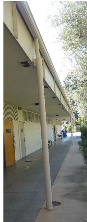
R2. Gutter and downspout.
