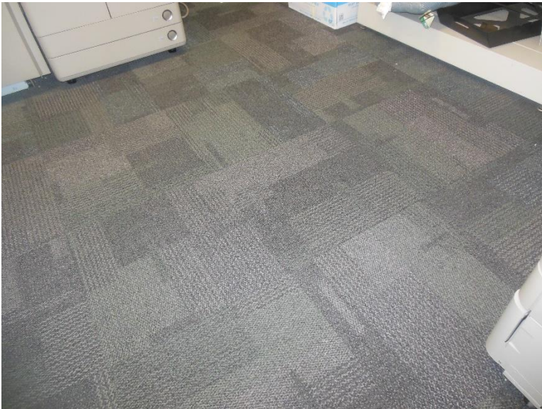
IF2. Copy room 10; carpet tile in good condition.
