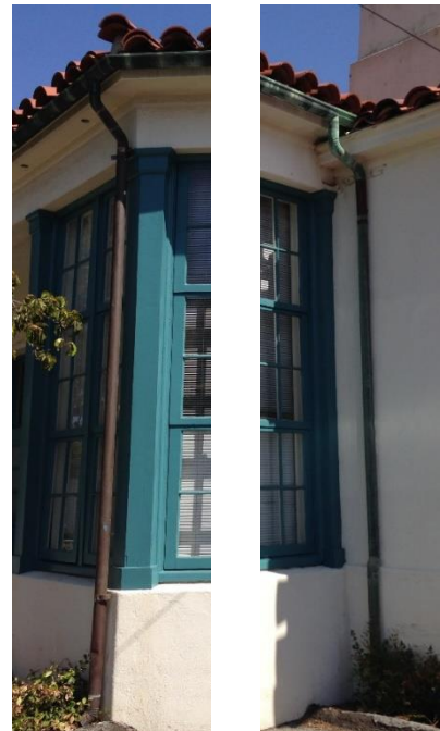
R2. Permanent buildings, copper gutters, downspouts and supports in good condition.
