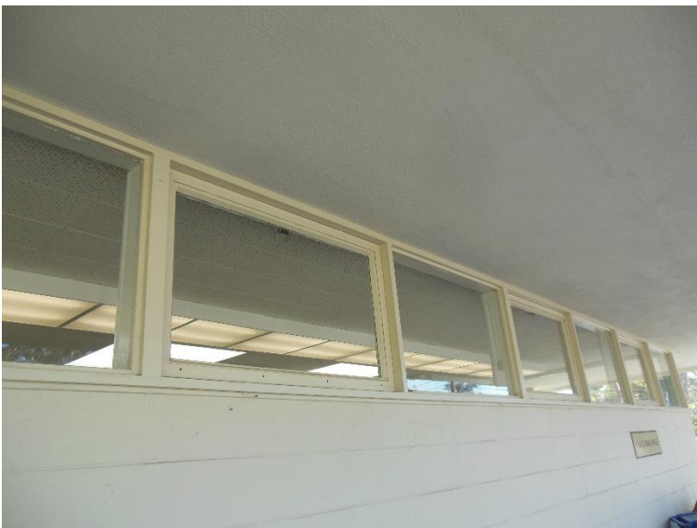
EW2. Exterior fixed wood windows; new paint.
