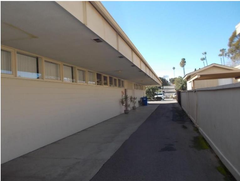
AE2. Exterior wall; painted CMU and wood, good condition.
