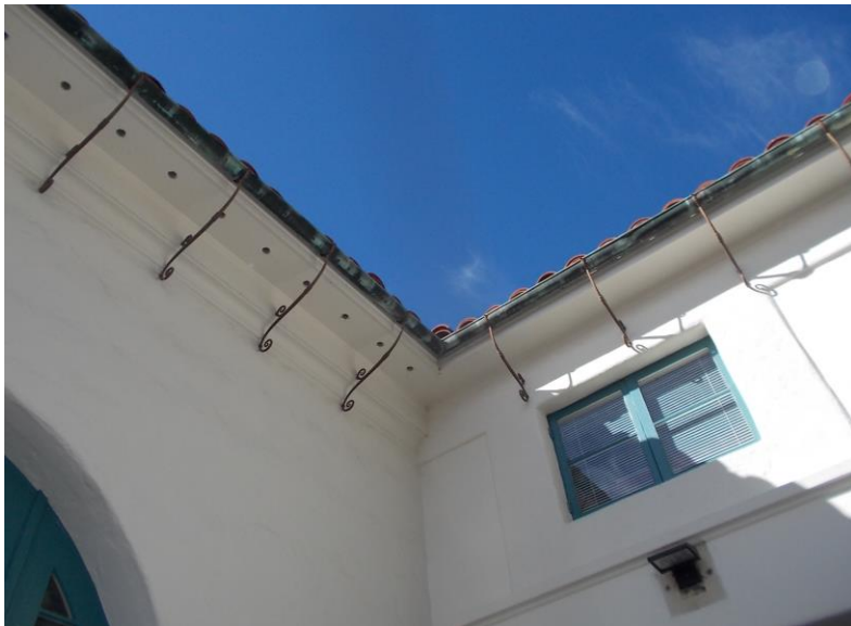
R2. Permanent buildings, copper gutters, downspouts and supports in good condition.
