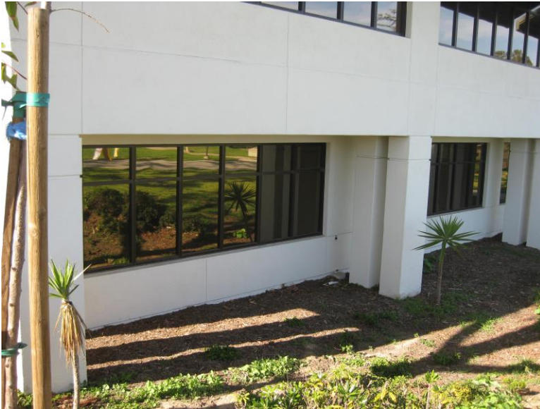
EW1. Exterior windows first level, in good condition.
