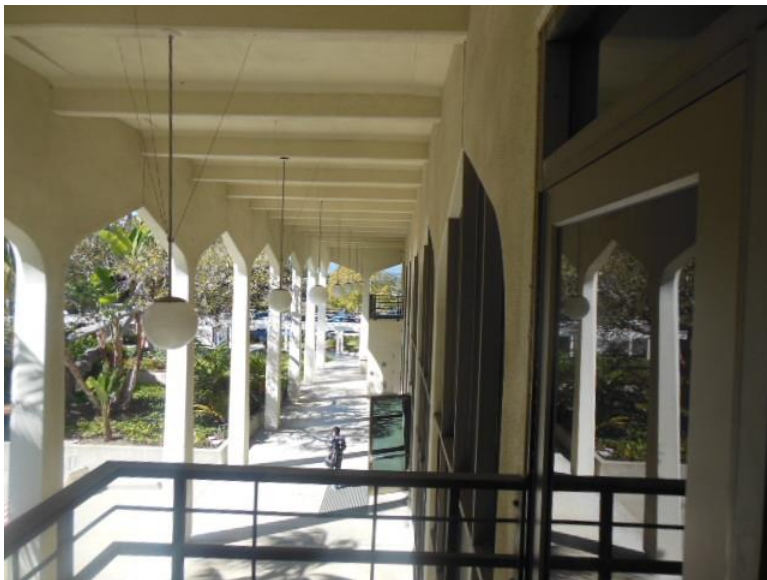
R2. Exterior underside of roof overhang.
