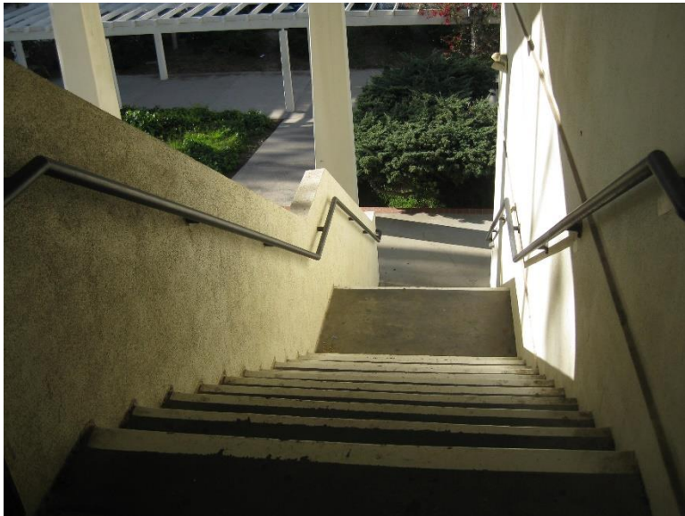
S4. Exterior northwest stair; stair nosing stripping faded, handrail heights and returns non-compliant.
