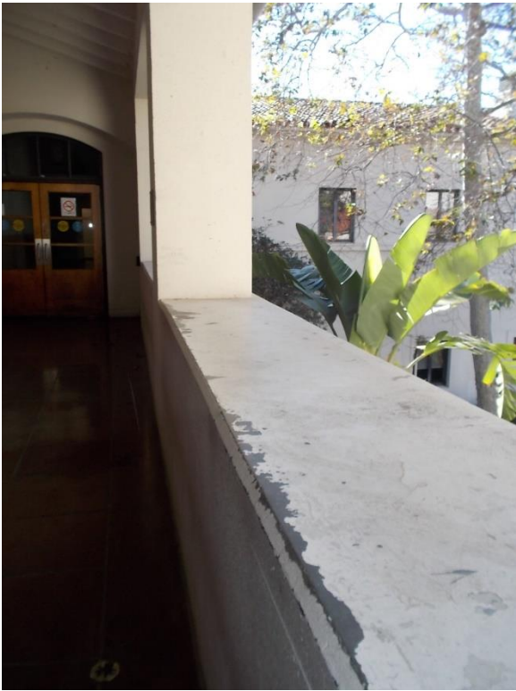
AE4. Northwest exterior walkway wall.
