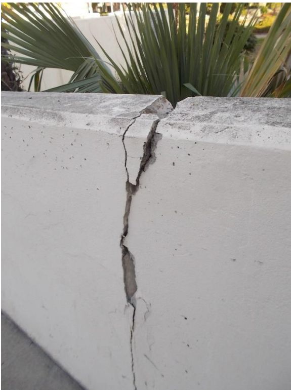
AE2. Northeast exterior ramped entrance walkway wall.
