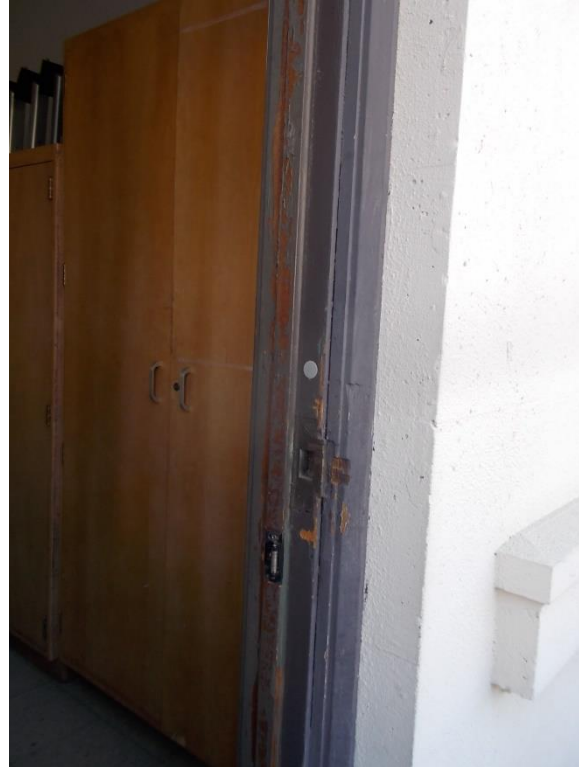
D2. 2nd floor exit door to stairs.
