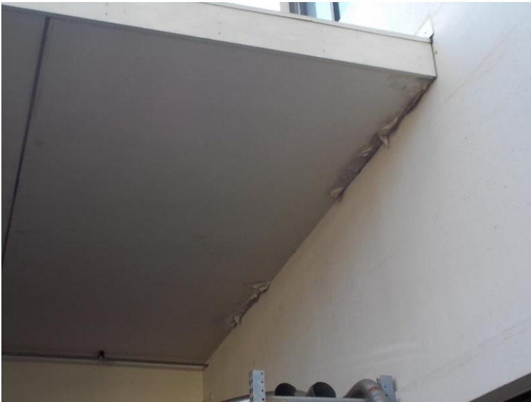
AE6. OE building, southeast exterior overhang.
