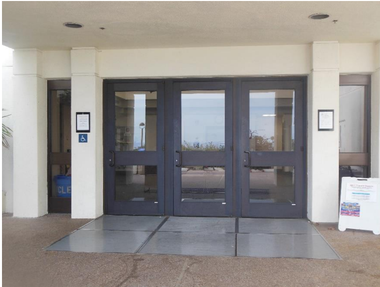
D1. Main Entrance; doors do not provide code required pull-side clearances, and wall mounted door identification signage.
