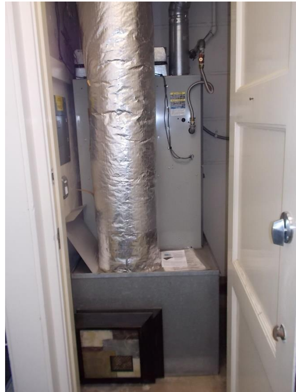
M3. Gas fired forced air heating units in mechanical closet adjacent space served, typical.
