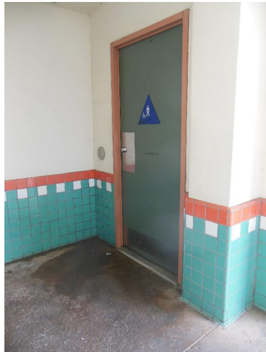
D5. Café restroom doors are missing wall mounted room ID signage. Low level access button for electronic door operator is required by code.
