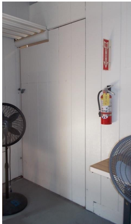
D4. Classroom patio; locked gate to exterior.
