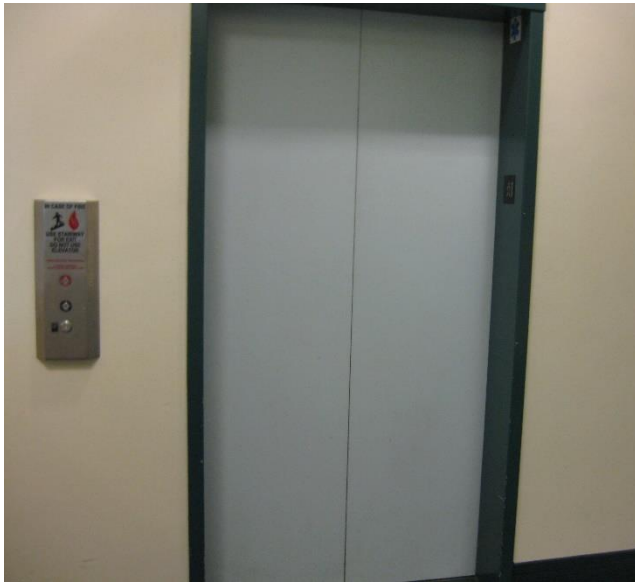
EV1. Elevator access to all floors.
