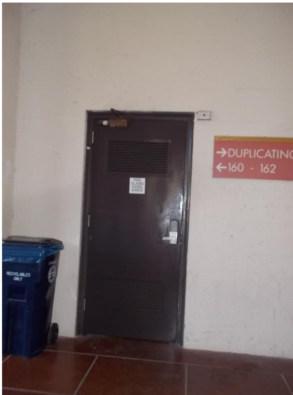
D3. Entry door to 1st floor Duplicating.
