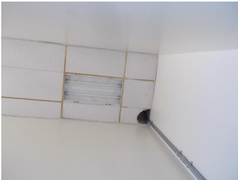
C2. OE stairway ceiling.
