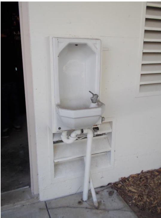
DF2. Drinking fountain in exterior walkway; hi-low fountains are not provided.
