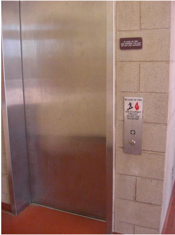
EV1. First floor elevator doors; missing proper signage.
