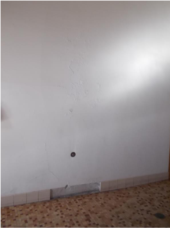
A13. First floor Men's Restroom.
