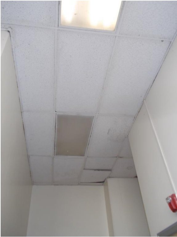
C3. OE second floor corridor.
