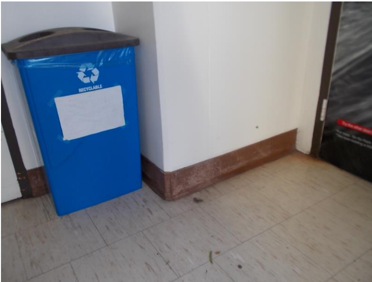
IF4. OE corridor second floor.
