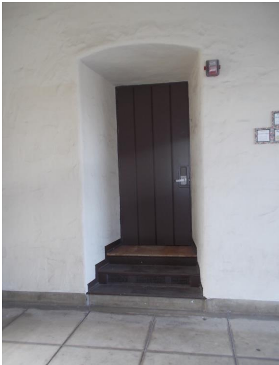
D4. Auditorium backstage door; pull-side clearances not met, stairs not accessible.
