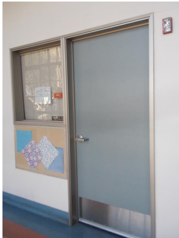
D4. Office door 2nd floor Health Occupations.
