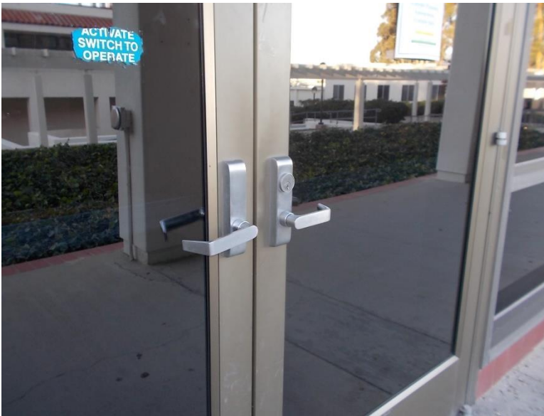
D4. South side entrance; doors require excessive force to open, electronic door opener lower-level push plate not provided and ISA sign not installed.
