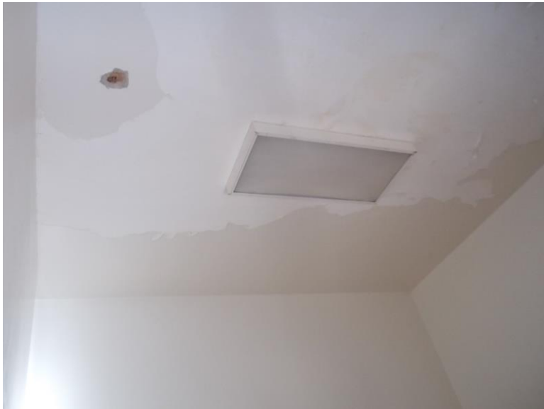
C1. First floor Women's Restroom.
