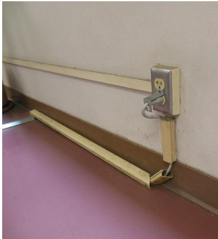
E5. Library, first floor; electrical duplex outlets, poor condition/installation.
