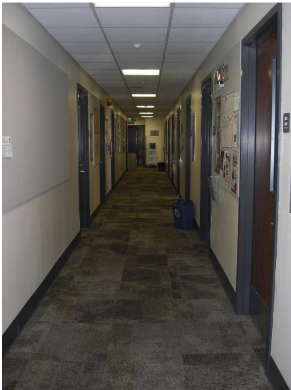
AI2. Third floor interior corridor walls; good condition.
