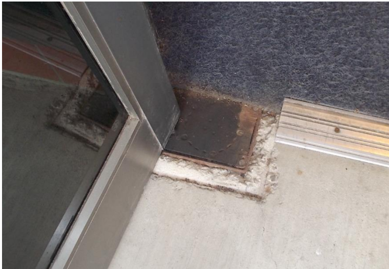
D6. West side entrance; door floor operator with exposed concrete.
