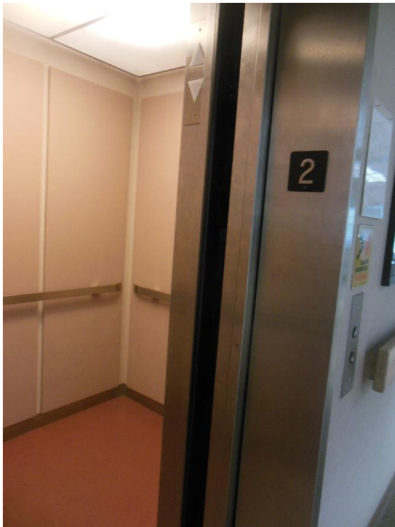
EV4. Elevator floor Braille sign at jamb.
