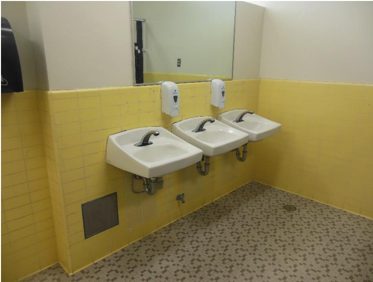
RR1. Women's Restroom; laboratories.
