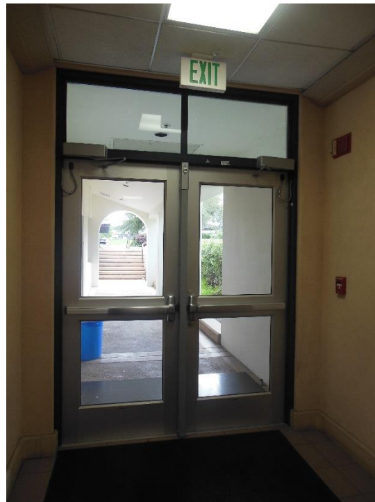
D8. Second floor corridor exit doors; missing wall mounted ADA exit signage and overhead exit signs are not illuminated.
