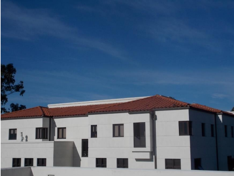
R3. Clay tile roof system, in good condition.
