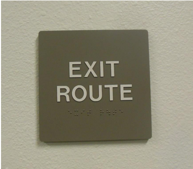
S1. Learning Center; ADA compliant exiting signage.
