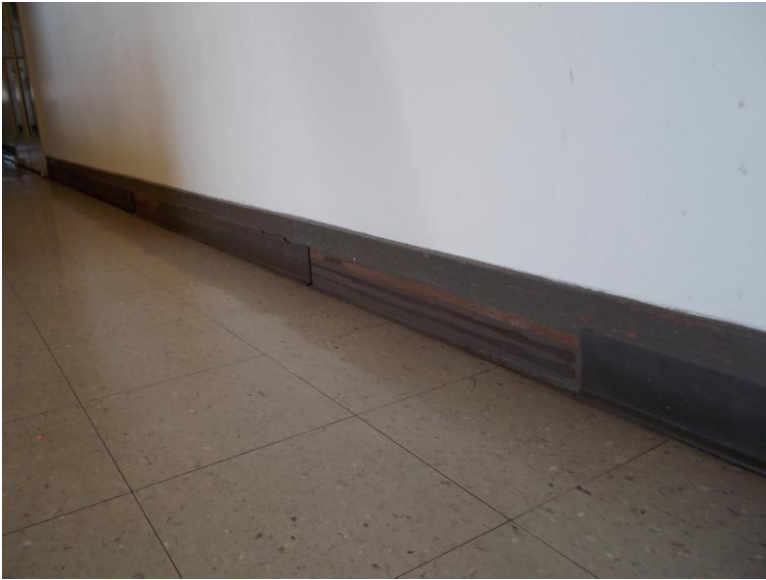
IF3. Southwest corridor second floor.
