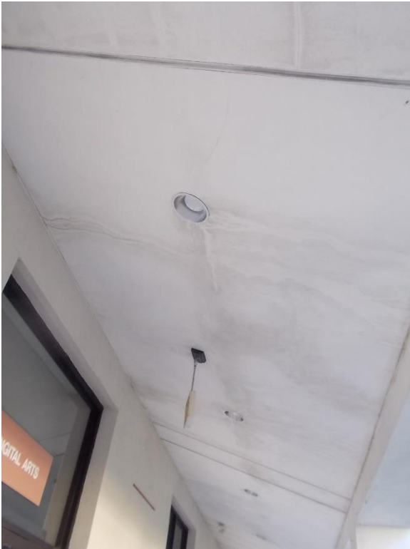
C4. Southeast corridor ceiling at offices.
