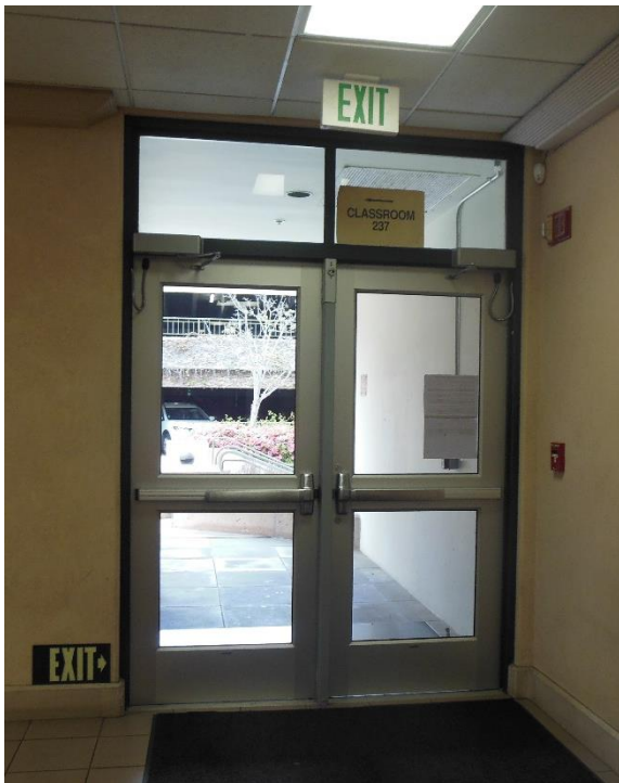
D8. Second floor corridor exit doors; missing wall mounted ADA exit signage and overhead exit signs are not illuminated.
