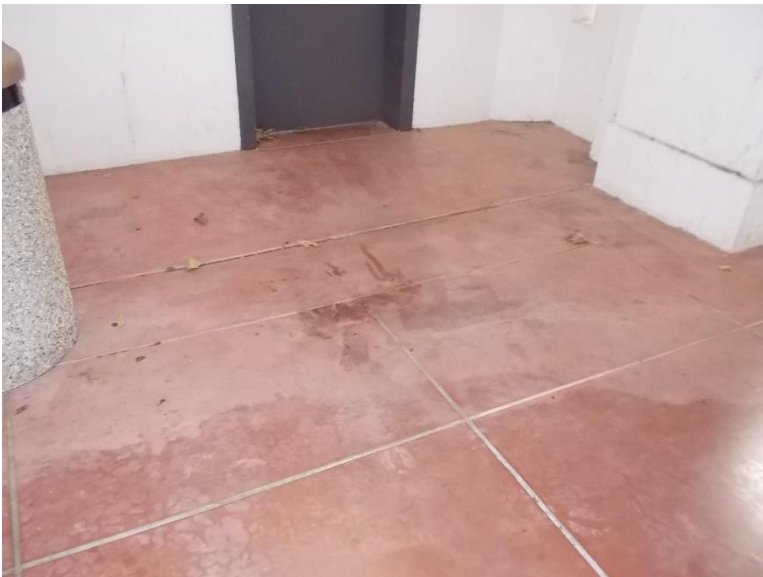
EF2. Northwest entrance to Elevator.
