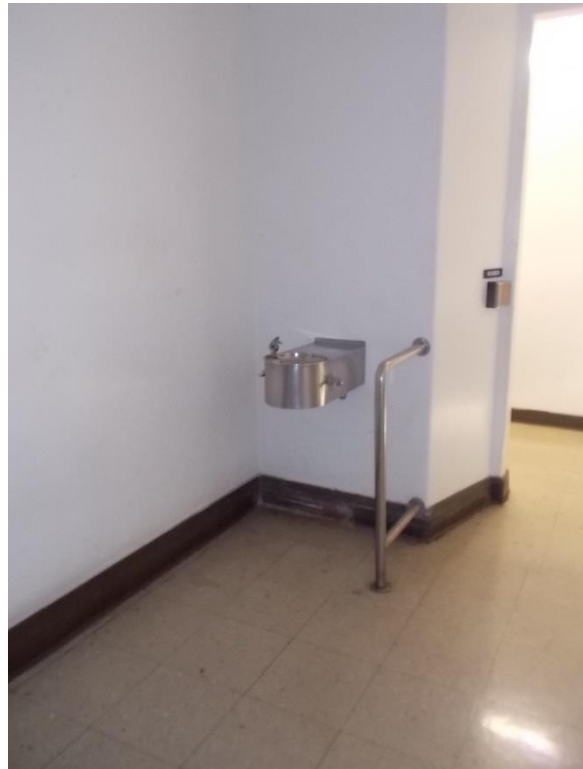
DF1. Second floor drinking fountain at restrooms.
