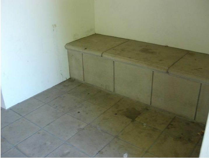
EF3. Third floor exterior concrete pavers and concrete stained finish.
