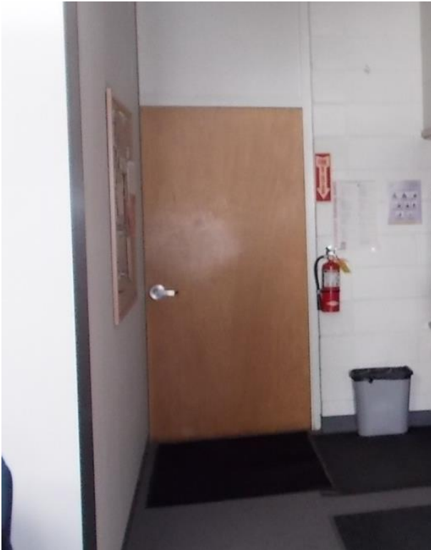
D1. Office 2; interior door.
