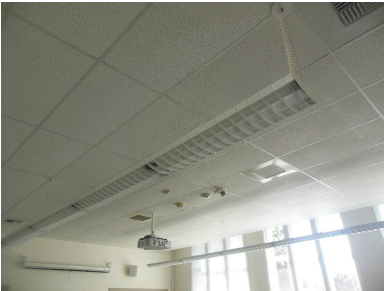
C2. Classroom; suspended ceiling system in good condition.
