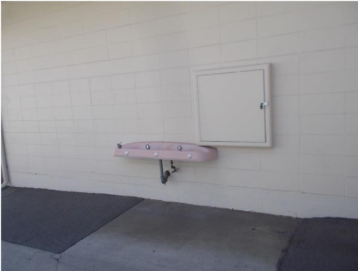
DF1. Drinking fountain in exterior walkway; hi-low fountains are not provided.
