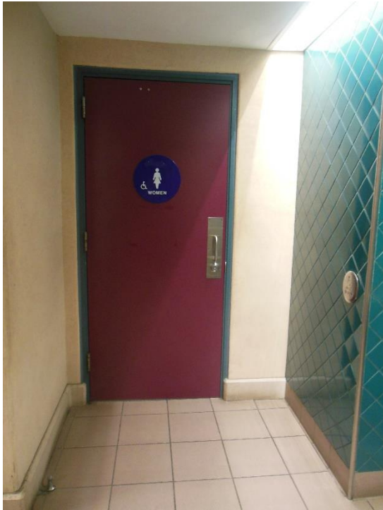
D7. Second floor restroom doors are missing wall mounted room ID signage. Low level access button for electronic door operator is required by code.
