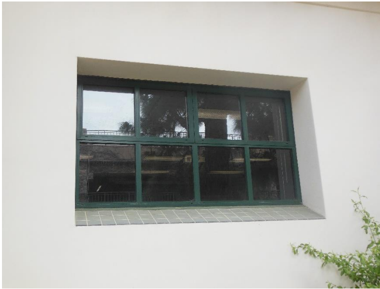
EW1. Aluminum framed lower floor windows and sill in good condition.
