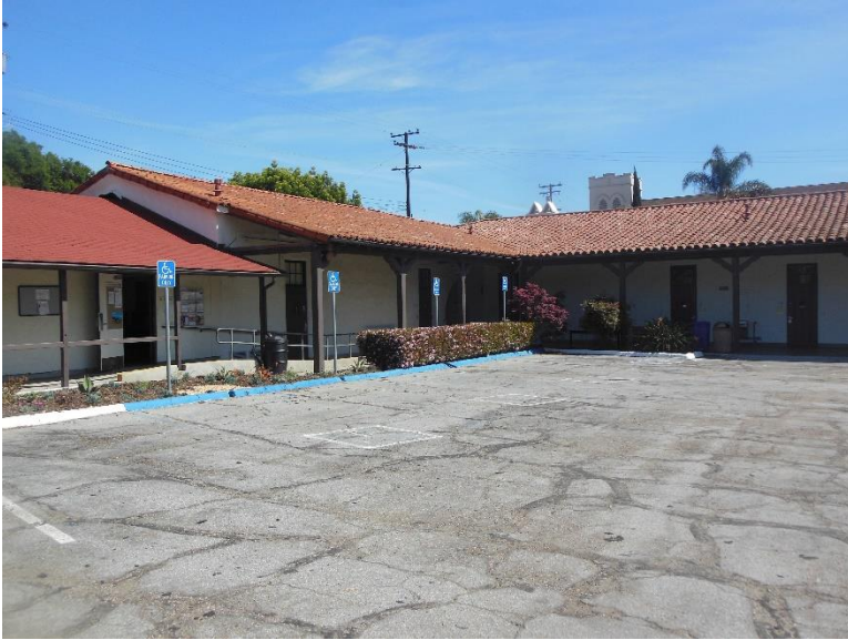
PT9. Accessible stall stripping degraded, layout not-compliant and no safe path from stalls to covered walkway.
