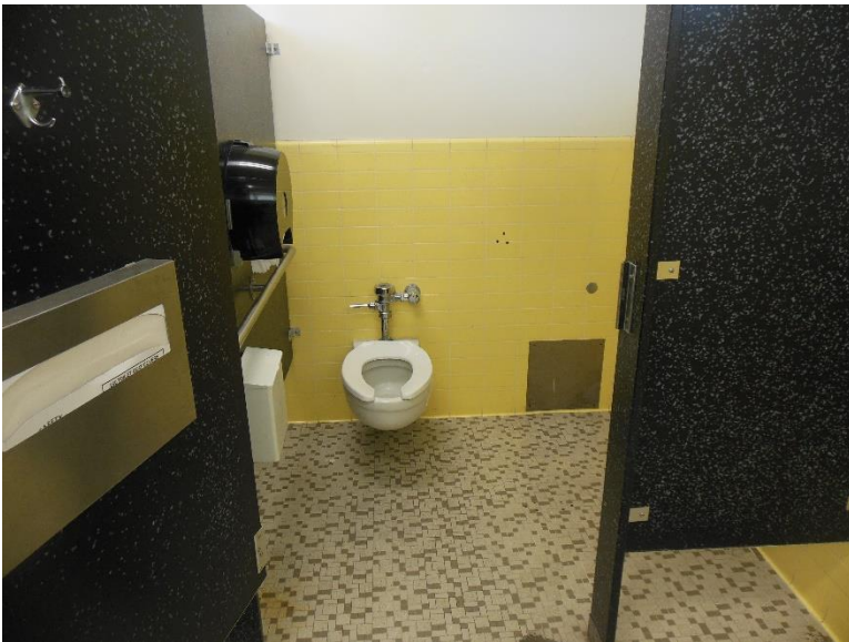
RR2. Women's Restroom; accessible stall, missing back handrail and stall size too small.
