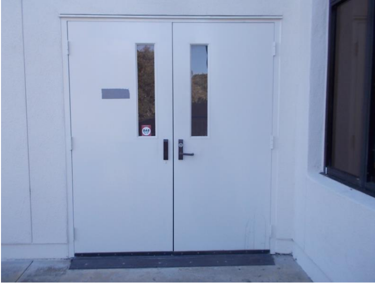
D3. Doors to stairs, at lower level; lacking code required wall mounted door identification signage.
