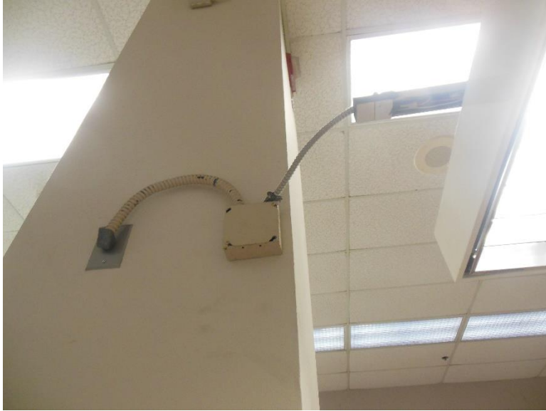
E4. Library, first floor; electrical light fixture connection.
