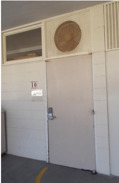
D1. Classroom 16; exterior door; fan in transom.
