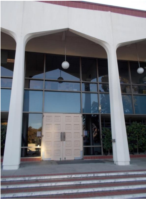
D1. East side entrance; doors require excessive force to open, electronic door opener lower-level push plate not provided and ISA sign not installed.
