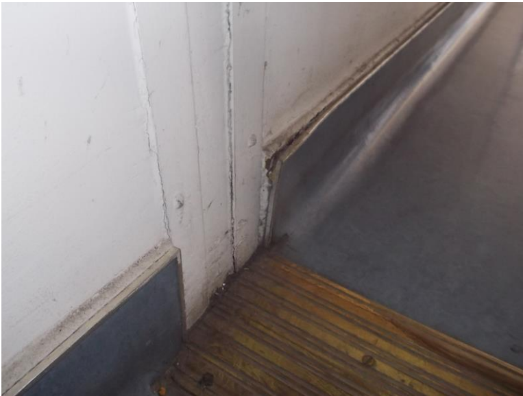
AI2. Second floor southeast interior corridor building joint.
