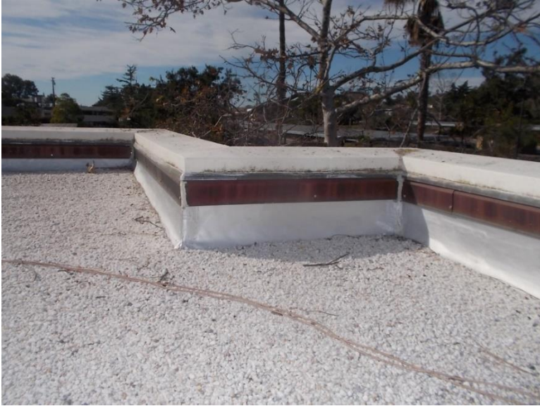
R3. Built up roof with plaster parapet.
