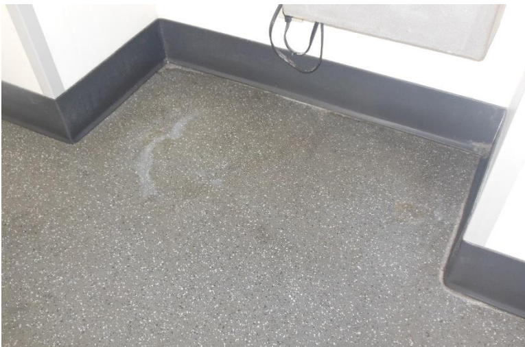
IF3. Lobby rubber tile and rubber base with water damage at drinking fountains.
