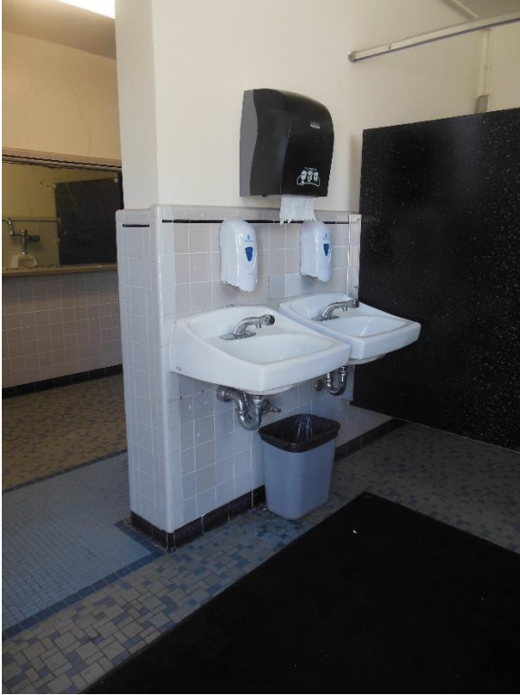
RR3. Men's Restroom; lavatories and fixtures.
