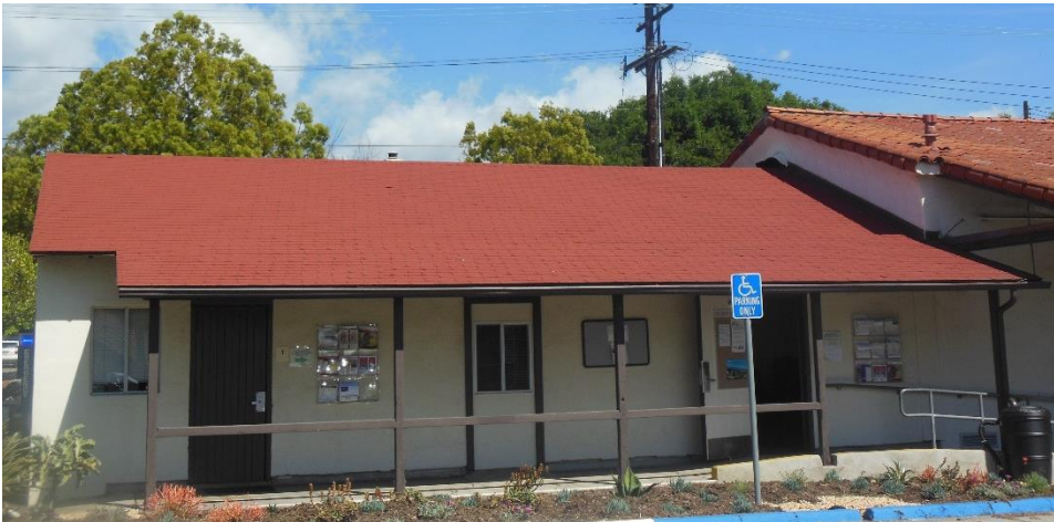
R4. Asphalt roofing over Offices 1, 2 and 3 in good condition.
