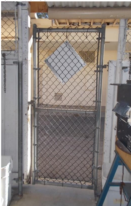
D3. Classroom patio; locked gate to exterior.
