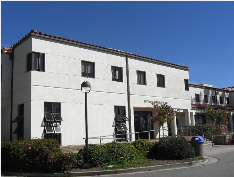
AE1. West facing entrance plaster wall.
