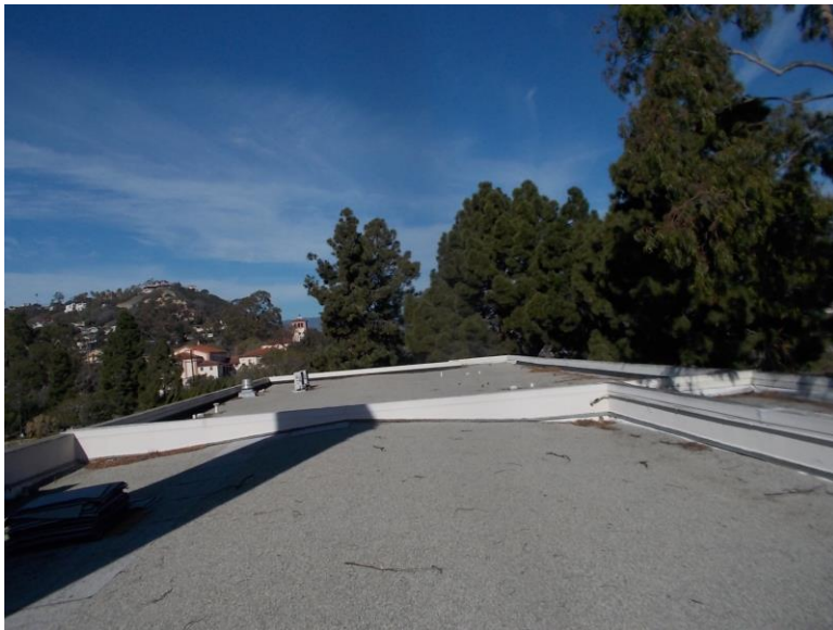
R2. Northeast wing built-up roof.
