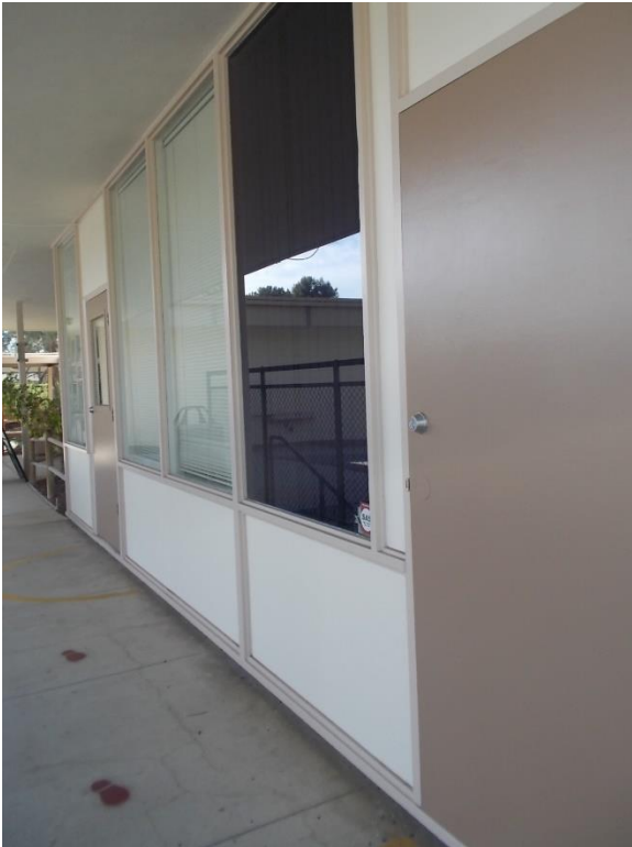
EW1. Exterior fixed wood windows; new paint.
