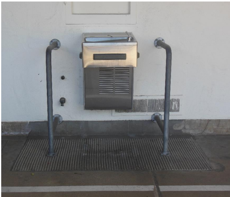
DF3. Drinking fountain in exterior walkway; hi-low fountains not provided
