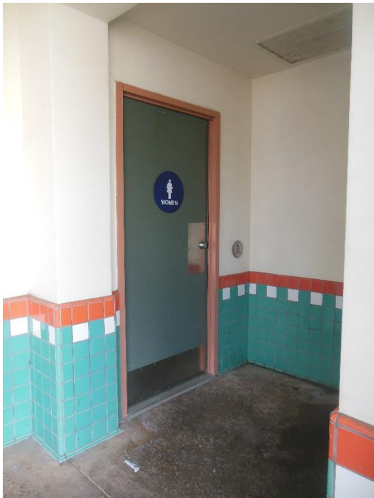
D5. Café restroom doors are missing wall mounted room ID signage. Low level access button for electronic door operator is required by code.
