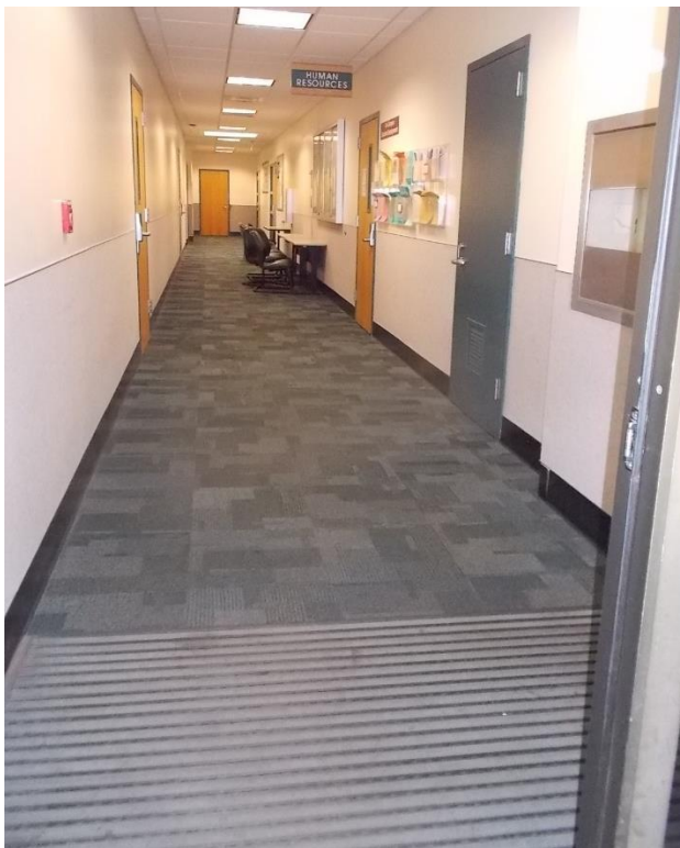
IF2. Second floor corridor; carpet tile, walk-off mat and rubber base in good condition.
