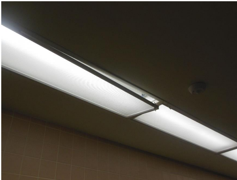
E3. Women's Rstroom 126; lighting fixture lens.
