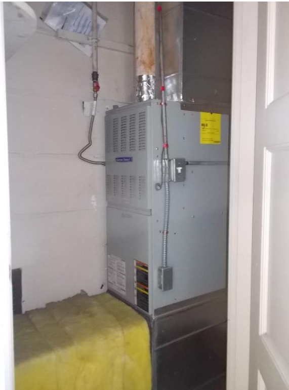
M3. Gas fired forced air heating units in mechanical closet adjacent space served, typical.
