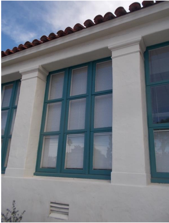
EW1. Exterior fixed wood windows; with new painted frames in excellent condition.
