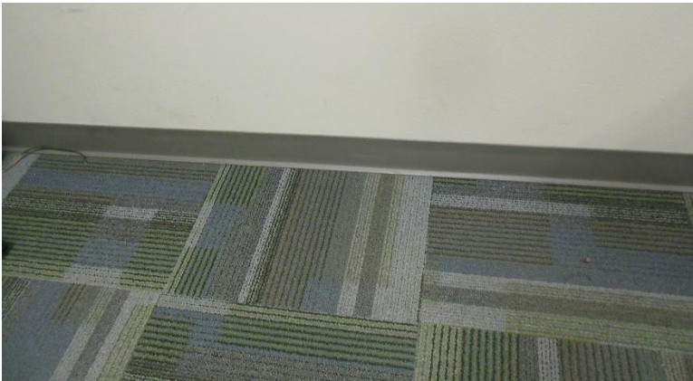
IF2. Learning Center carpet tile and rubber base in excellent condition.
