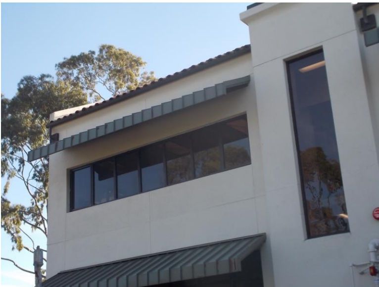
EW2. Exterior upper level windows, in good condition.
