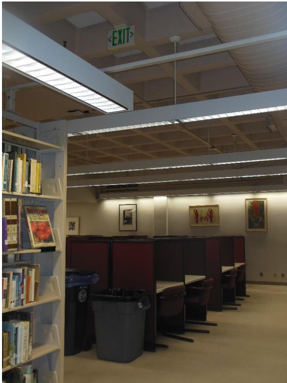
S4. Library, lower level; exit sign not illuminated, and excessively high for visibility.
