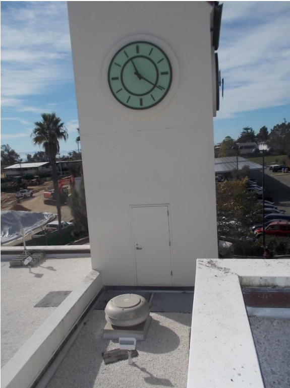
R4. Clock tower at plaster parapet.
