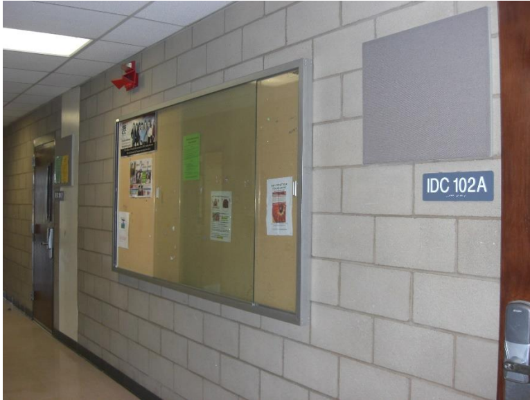
AI1. First floor interior corridor CMU walls; good condition.
