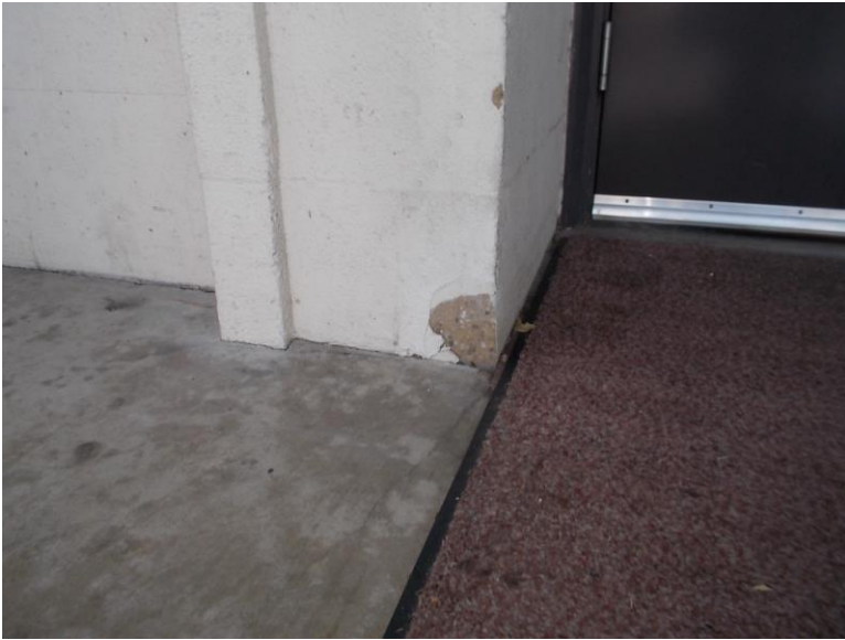
AE3. Northeast exterior entrance column.
