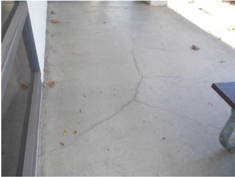
EF3. Southeast OE exterior corridor.
