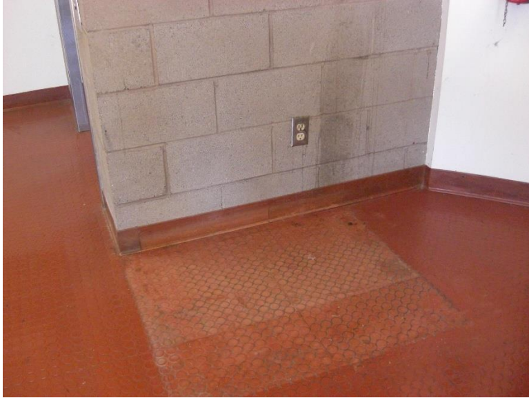
IF3. First floor exit passageway at stairwell enclosure by elevator. Damaged rubber flooring and resilient base.
