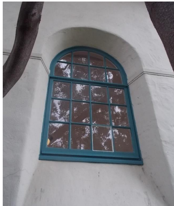
EW4. Exterior fixed wood windows; with newly painted frame in excellent condition.
