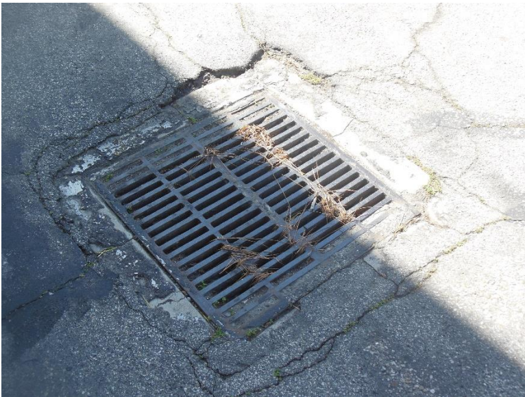
EF4. Drainage catch basin on parking lot with degraded surrounding asphalt materials.
