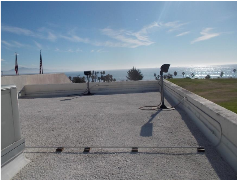
R4. Built-up roof system in good to excellent condition. Flood lights serve to light the walkways and plazas below.
