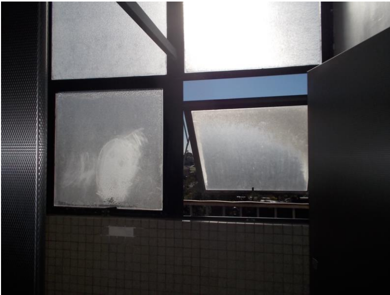
EW5. Second floor Women's restroom.
