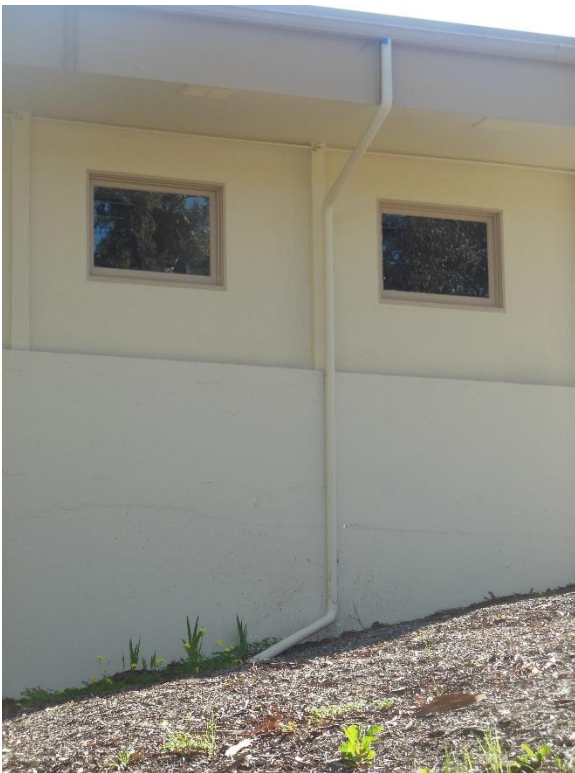
AE4. Exterior painted concrete and plaster.
