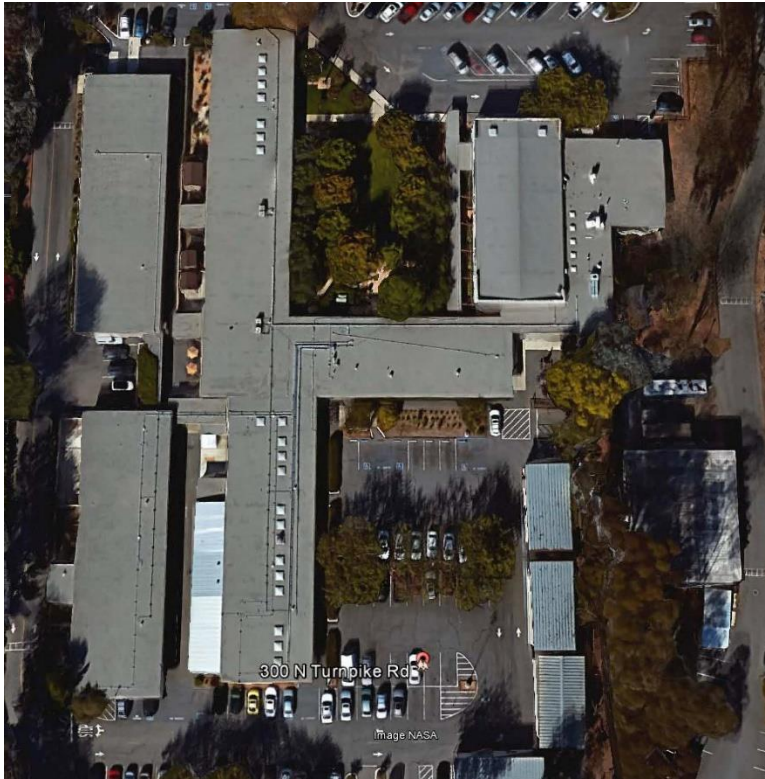
R1. Overall site; roofs.
