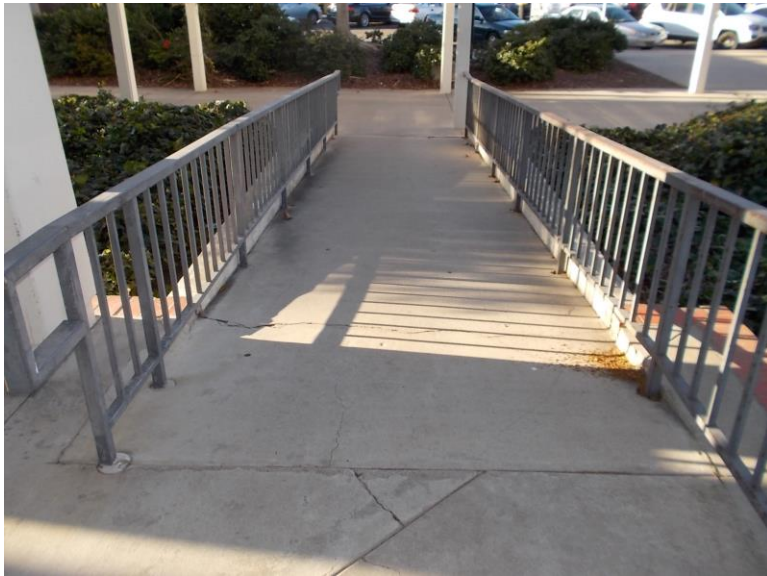
PT1. Exterior north ramp; non-compliant ramp. Handrails heights are too short, gripping surface is too wide, and ramp has excessive running slope. ADA directional signage is not provided.
