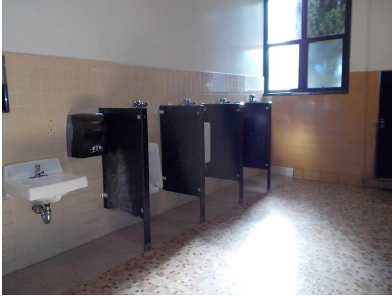
RR3. Mens restroom, first floor southwest wing.
