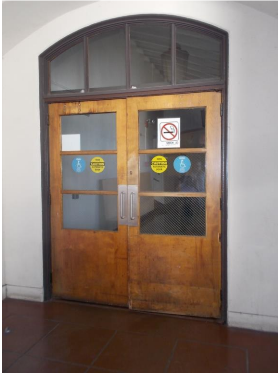
D1. First Floor entrance doors near elevator.
