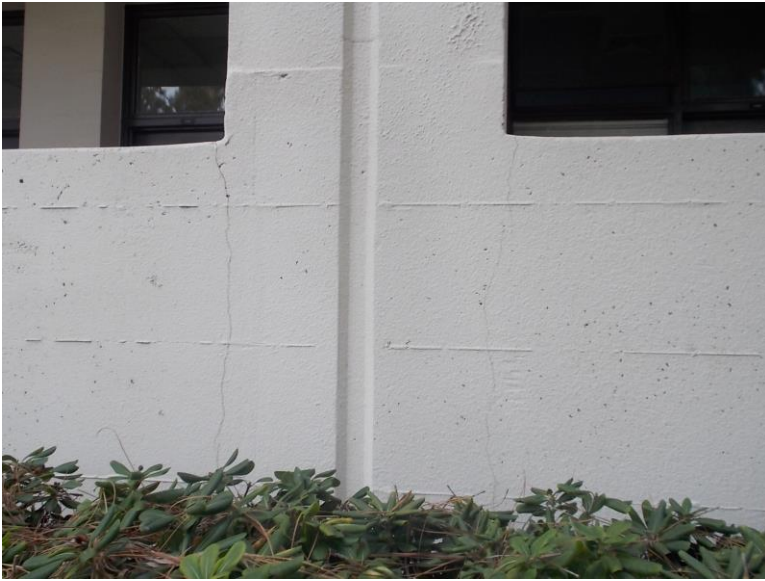
AE1. Northeast exterior walkway wall.
