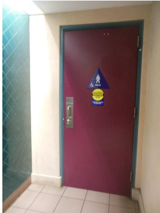
D7. Second floor restroom doors are missing wall mounted room ID signage. Low level access button for electronic door operator is required by code.
